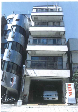
▲3号館 Annex Building
